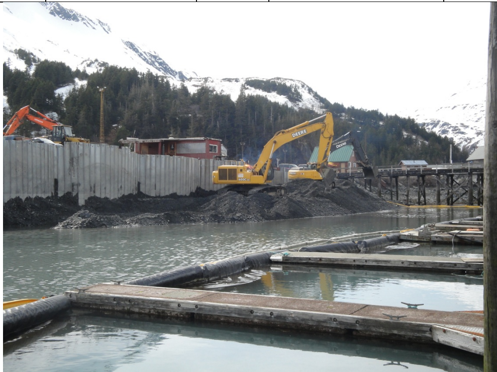
Whittier Harbor Dredging project
