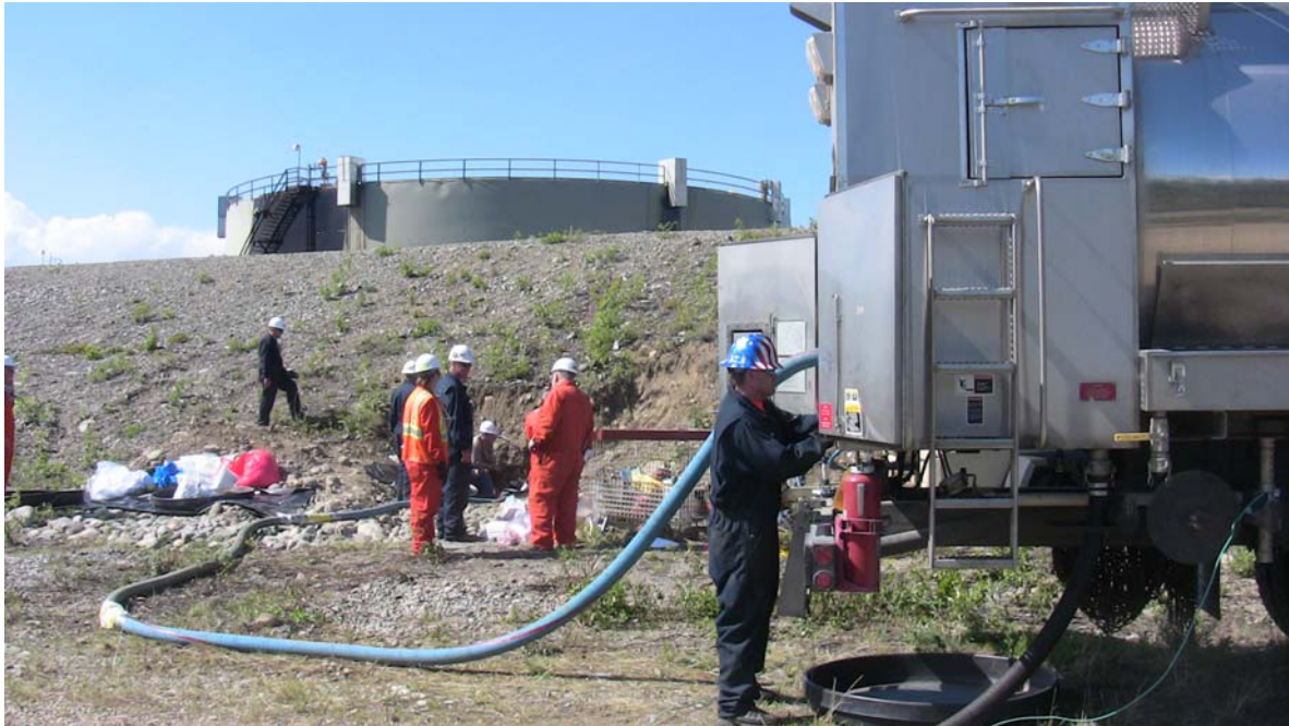
APSC crew pumping oil from the containment drainage pipe on May 27. (APSC photo)
