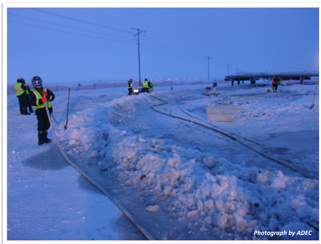
The day-shift crew building an ice berm around the spill site in preparation for steamer tactics.
