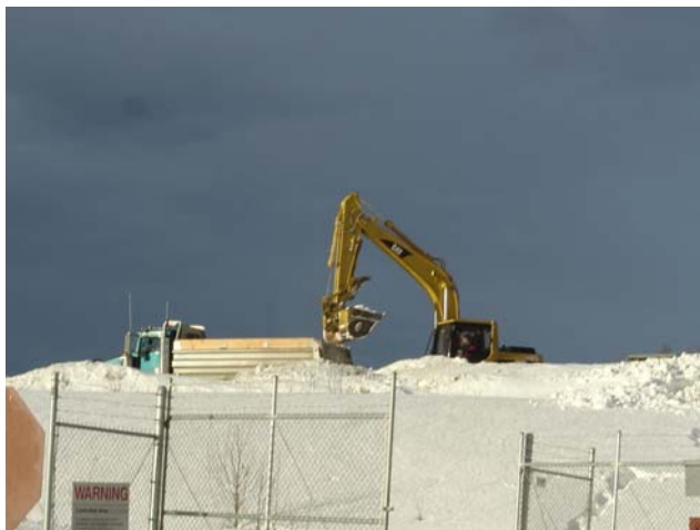
Fuel contaminated snow being loaded into a dump truck for transport to disposal site.
