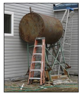
The set up of this tank makes it very vulnerable to damage from an earthquake or a flood.
